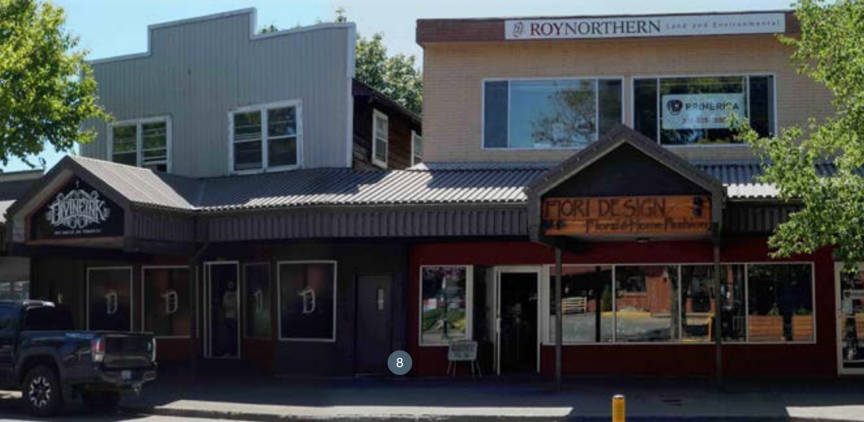
Historic facades and architectural elements behind canopy and renovations
