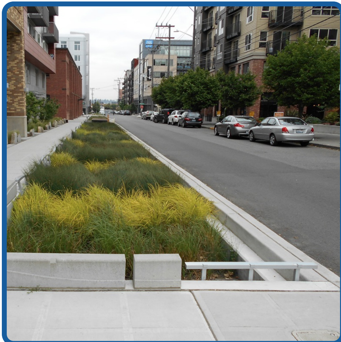
GREEN INFRASTRUCTURE (BIO SWALES)
