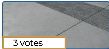
SAW-CUT & SANDBLASTED CONCRETE
