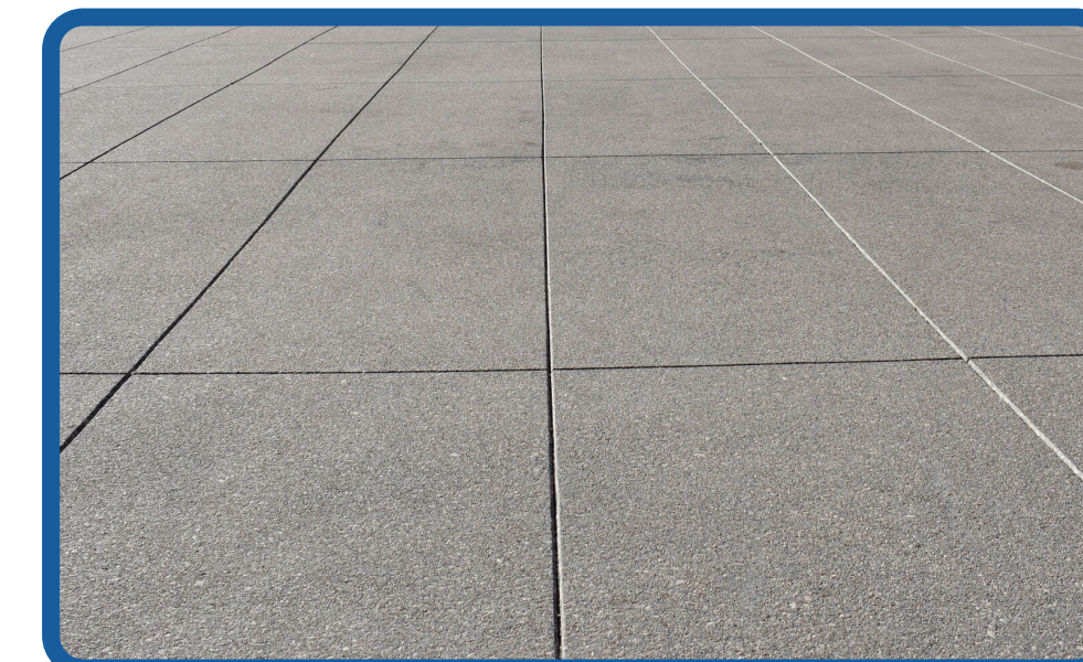
CONCRETE WITH SAW CUTS
